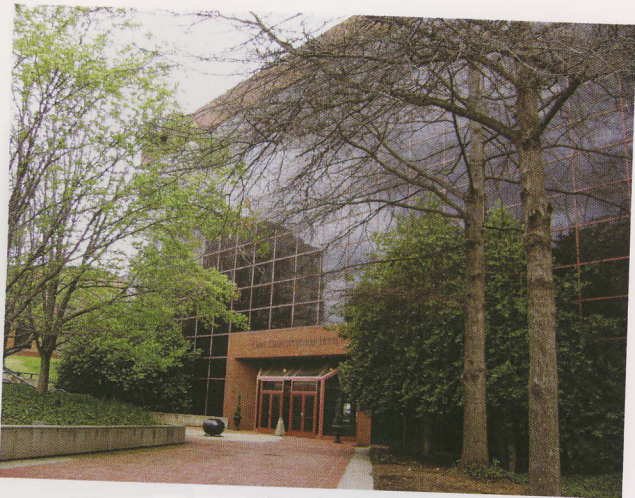
Principal façade on Main Street
