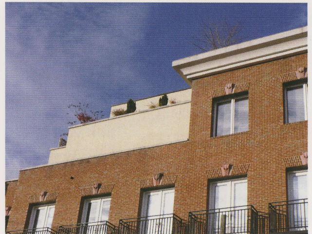
The Terraces, detail of terraced rooftops, Water Street Side, 1997
